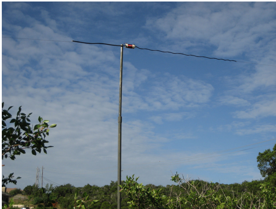
Figure 6. Plastic pipe support and resonant LC circuits at the antenna center.
