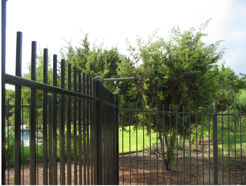
Figure 7. Antenna spring used to tie the 46 ft leg to the fence.
